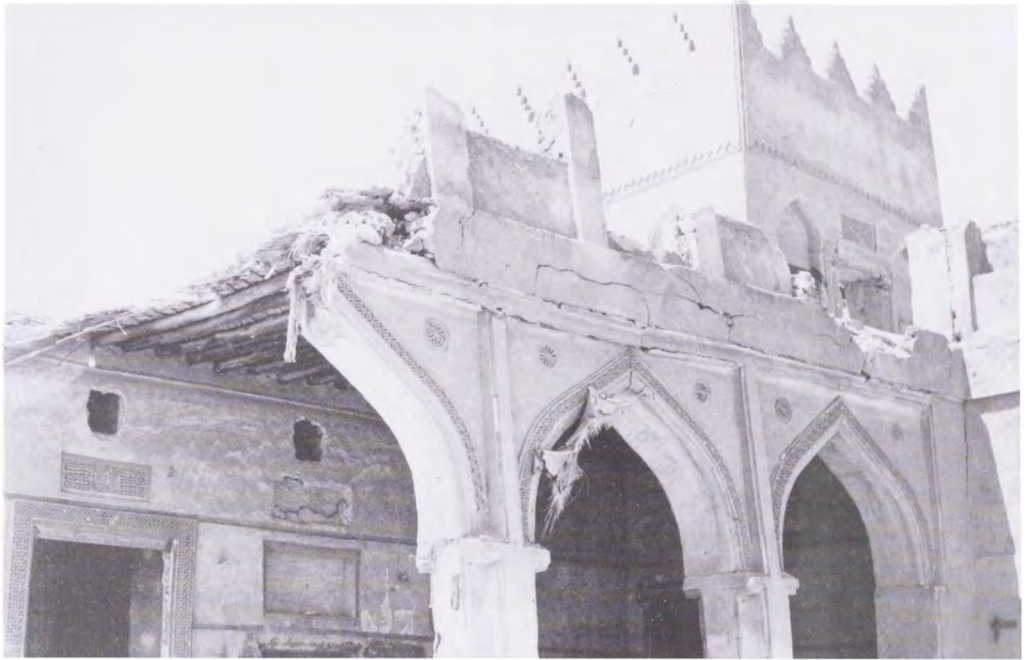
(Fig. 9) : Sheikh Abdullah's residence before restoration.
